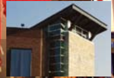
A precast concrete tower incorporates conventional masonry and glass, plus custom exterior finishes and touches. Photo: Tindall Corp.
